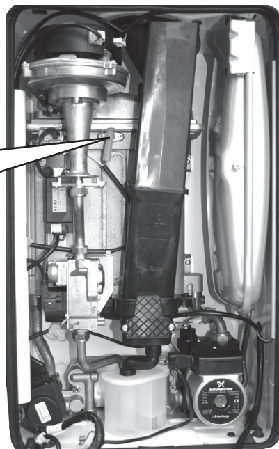
Flame Detection Electrode
