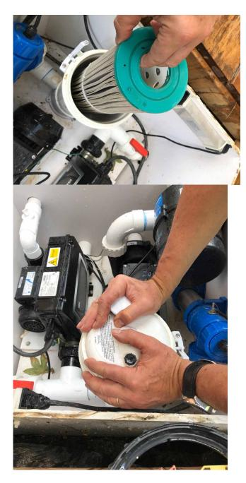
Replace the lid and carefully apply downward pressure ensuring that the lid is properly sealed. Apply black screw lid. If it is not properly sealed you will notice it is dribbling once the water is again introduced into the filter chamber.
