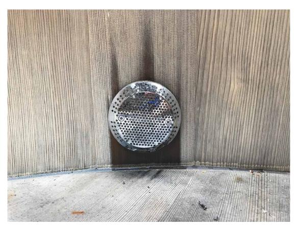
[It maybe necessary to do this clean these inlets every couple of weeks if the house is booked often, you will have to jump in and clean them by hand.! }When the tub is empty is a good time to change the filter. Once empty you can just take it out and replace before refilling. Refill and loosen the small black valve on top of the filter holder.
