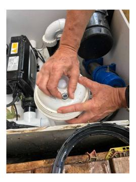
this will hiss as the water comes in and then when water comes out of it, tighten and close. This prevents air being stuck in system.
