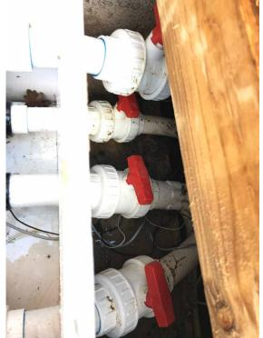
2.Open 1x pipe valve inside power plan box( turn red lever in line with flow to
