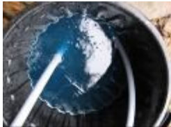
Fig 25 Slinkies Purged of Air
